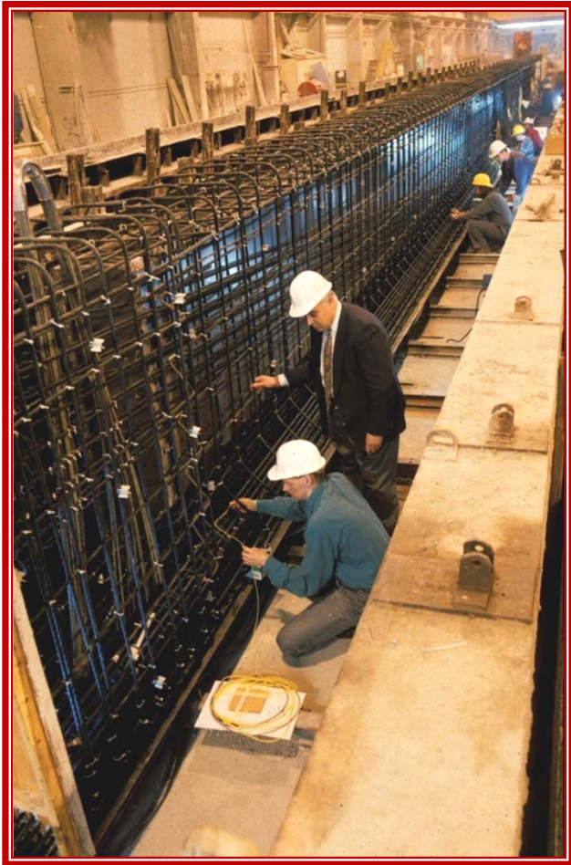
Instrumentation of the girder before casting
