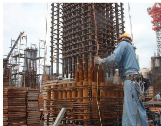
Slim Sleeve for connecting rebar cage
