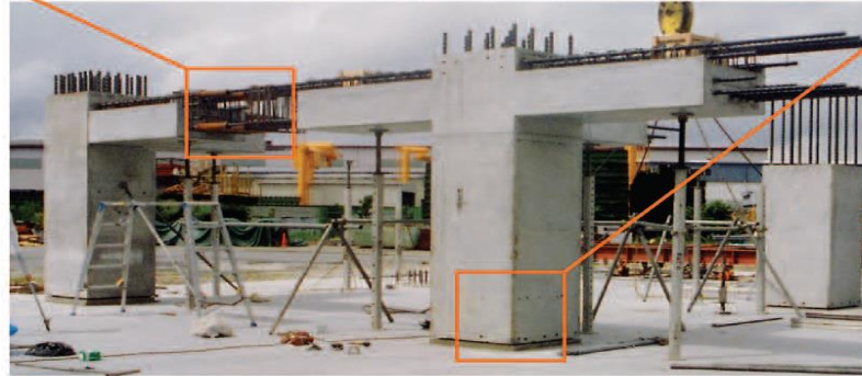
Super UX, NX II Sleeve for Precast column
