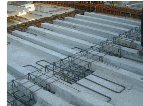
Half PCa Slab with Prestressing
