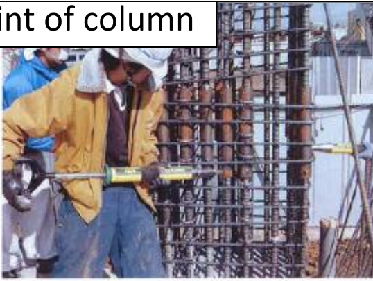
Mechanical joint (Cast-in-situ)
