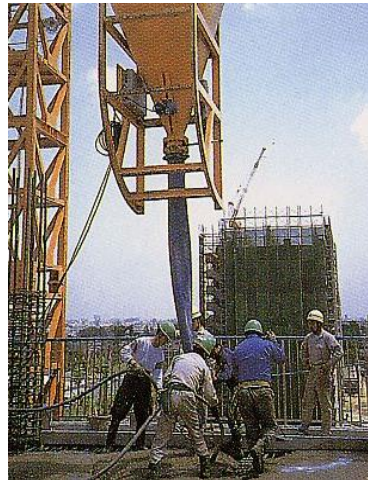
⑤ Casting Concrete
