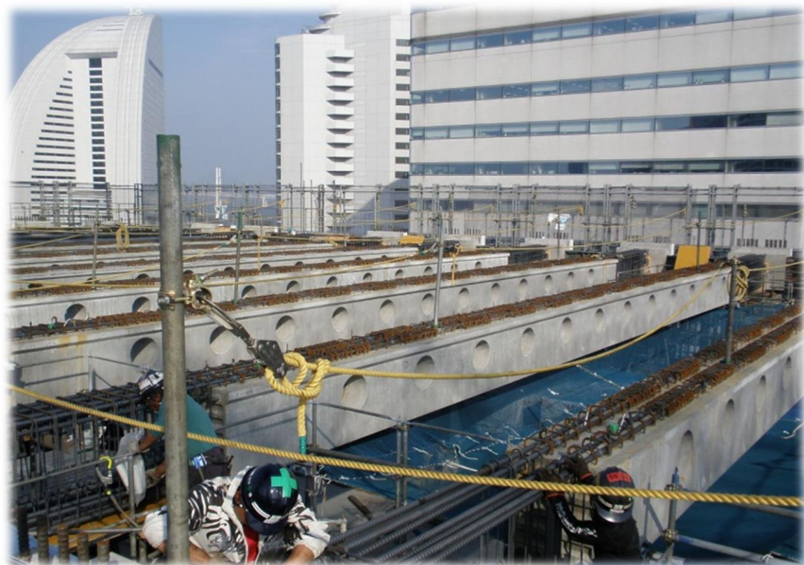
Prestressed concrete beams
