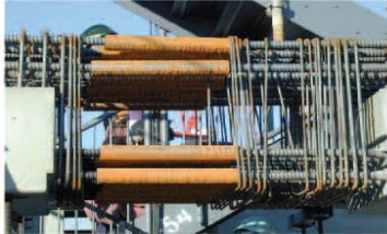
Slim Sleeve for connecting Precast beams
