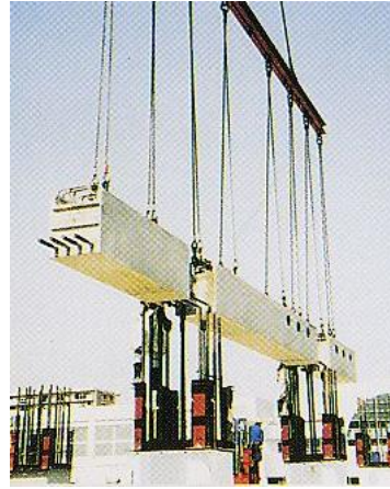
② Placing of PCa Girder
