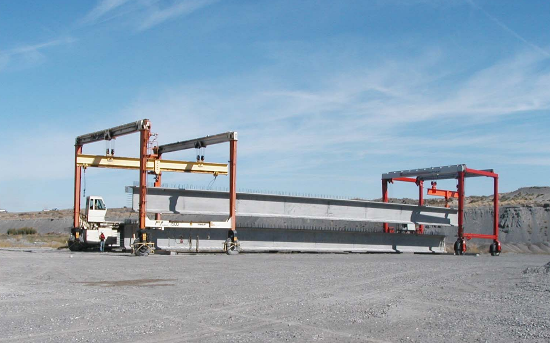
Washington state 2.1 m deep, 47.2 m long for construction over the Yakima River
