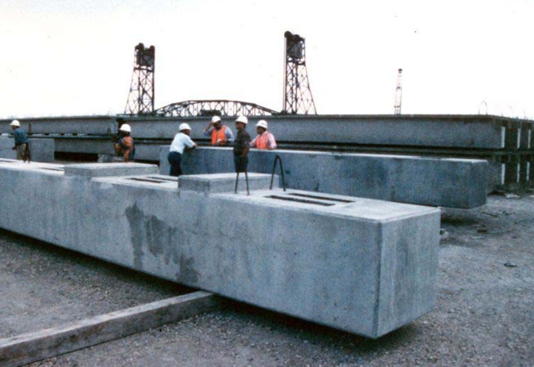
Precast Pier Cans
